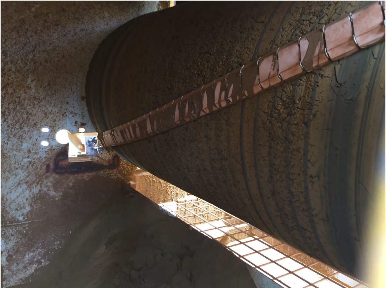
Figure 8: Rigid cleaner tips are inefficient on severely pitted belts.
