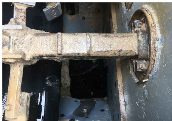
Image: Previous Wear Liner Install (after 3 months service)
