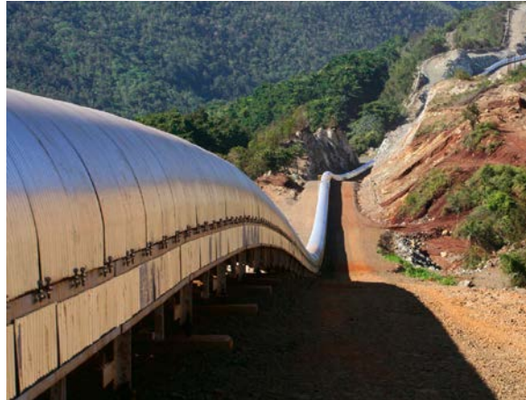
Steel belt covers on an overland conveyor
