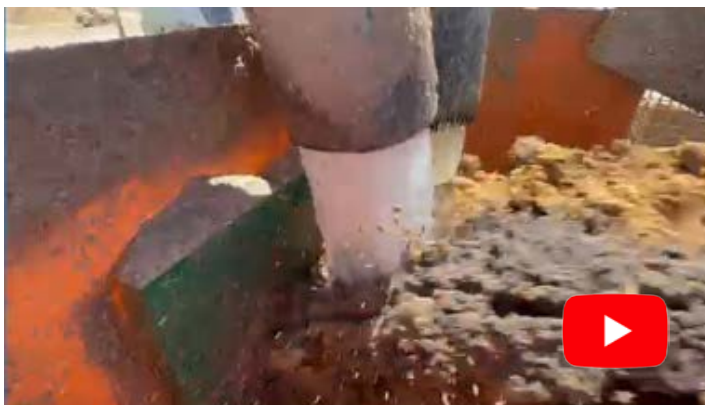
After Photo / Video: K-Redi-Liner® Polyurethane installed at the head discharge chute.
